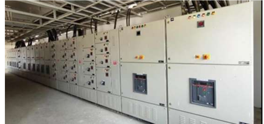
LT PANEL INSTALLATION WORK
