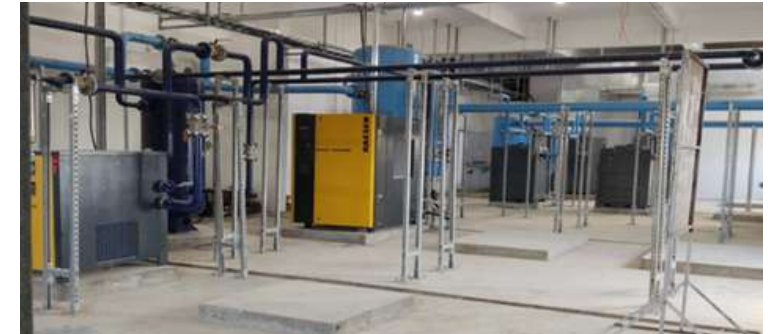
Compressor Installation Work
